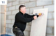
Step 1 Place boards into position around the tray to check fit. Run two beads of MEGA Strength adhesive onto the back of **No**More**Ply**.
